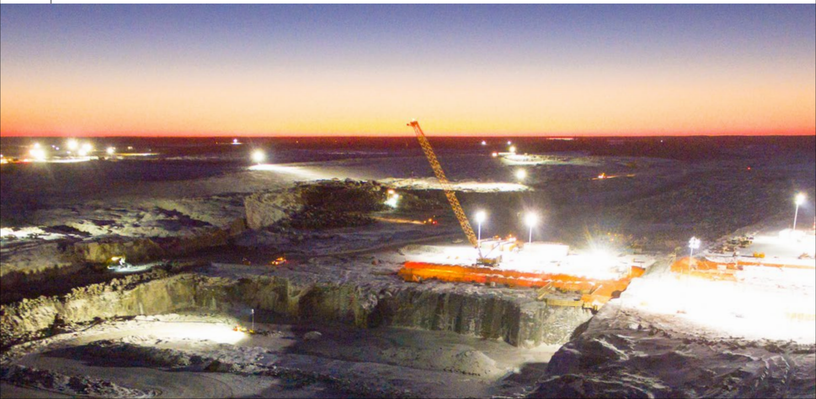
Keeyask Generating Station, Manitoba, Canada
