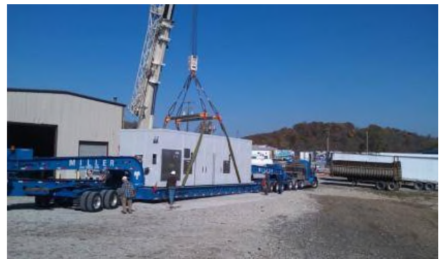
Figure 4. Echogen EPS 100 Process skid (left) and Power Skid Right (Courtesy Echogen Power Systems and Dresser-Rand)
