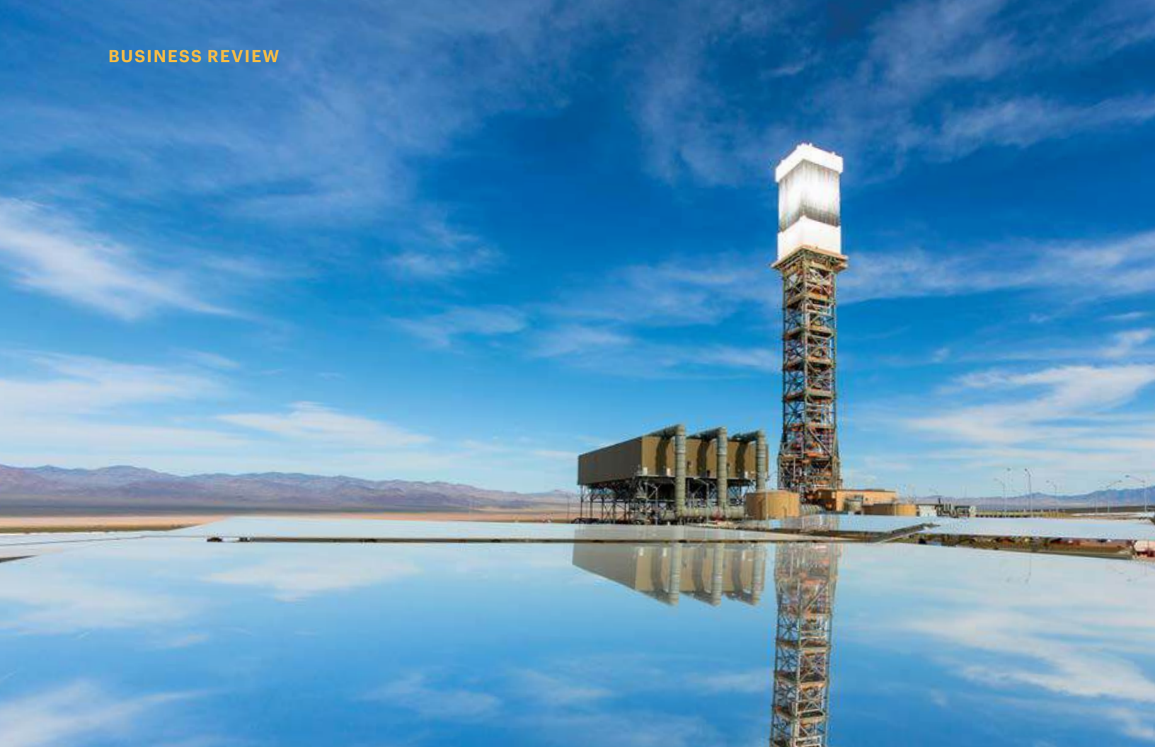
▲ Ivanpah Solar Electric Generating System California, USA
