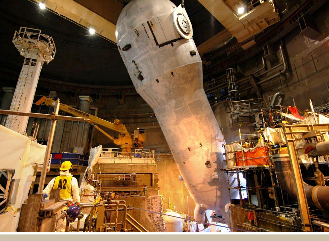
plants is to cut a hole in the wall of the containment building that houses the reactor, because the maintenance doors are too small and there is little room to maneuver equipment inside.
