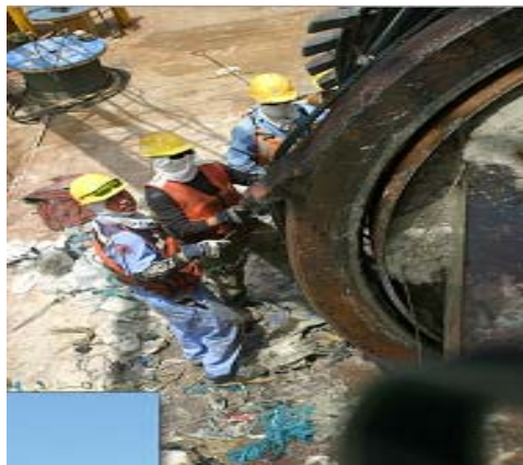
Cleaning trash collected on dredge intake, Port of Umm Qasr
