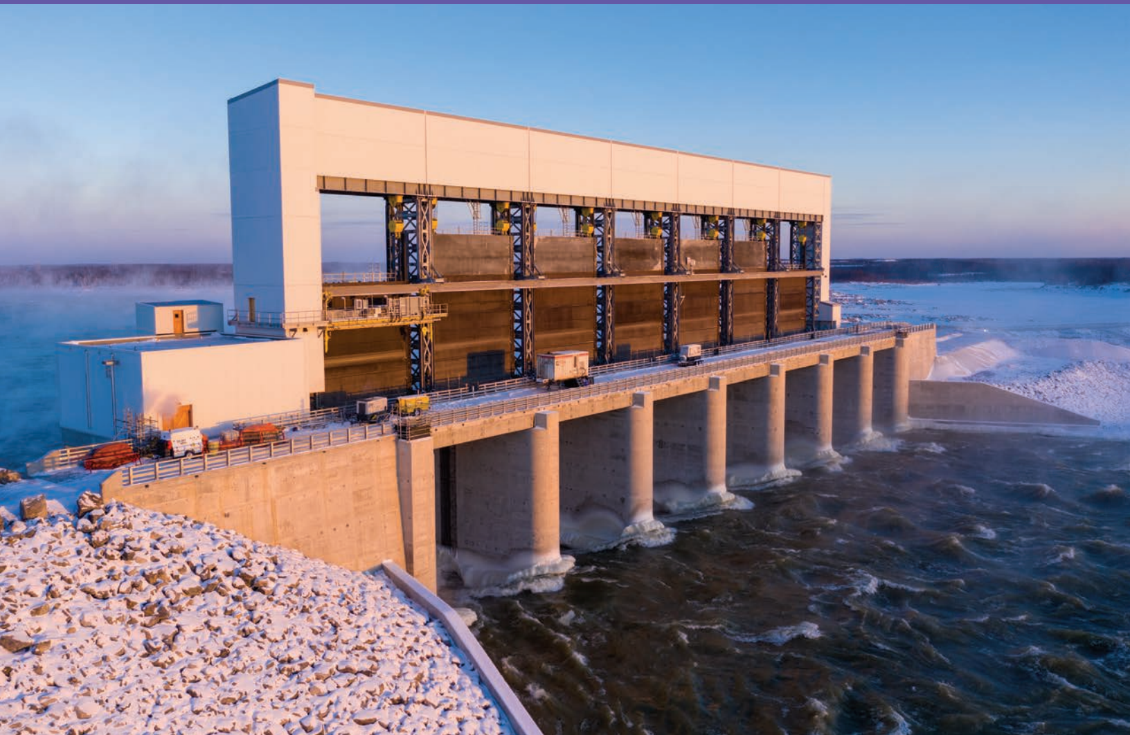
▼ Keeyask Generating Station, Canada
