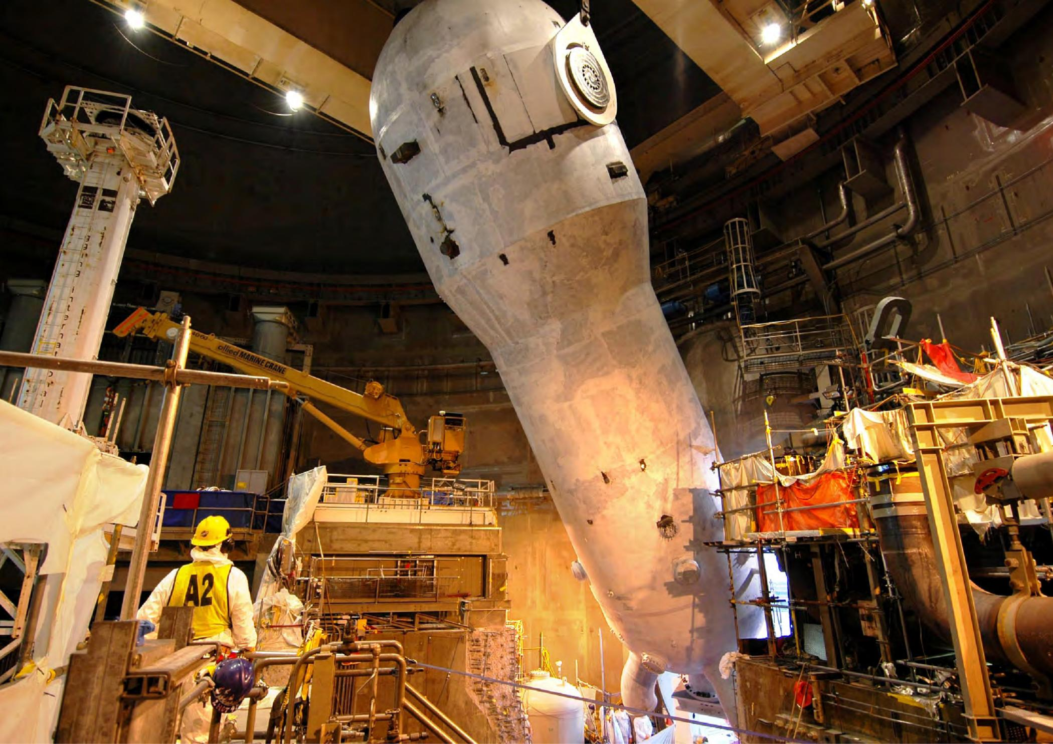
plants is to cut a hole in the wall of the containment building that houses the reactor, because the maintenance doors are too small and there is little room to maneuver equipment inside.
