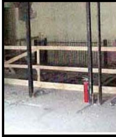
Picture of a leading edge properly protected with a hard barricade.
