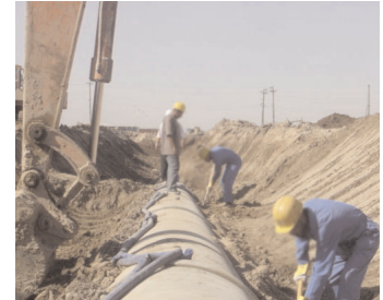
Treated water pipeline backfill at a community in central Iraq
