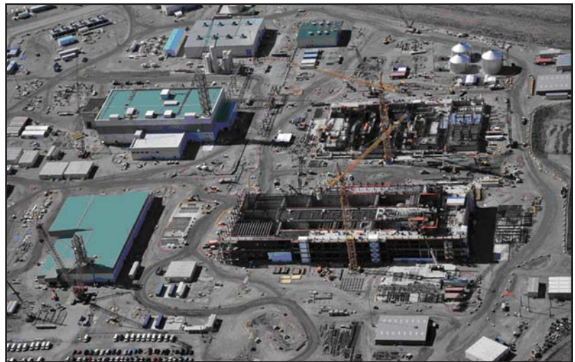
Figure 1. Hanford Waste Treatment Plant Facilities, Washington State
