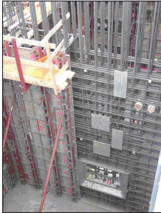
Figure 7. Rebar at Shield Window (Note Multiple Layers of Reinforcing)
