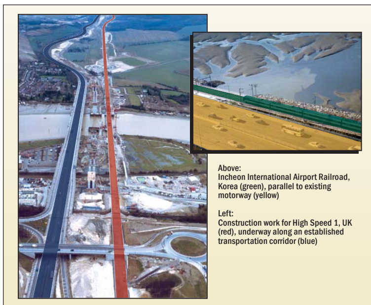
Figure 5. Examples of Using Existing Transportation Corridors for Railways
