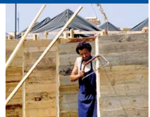
A local worker helps with the construction of the temporary camp.
