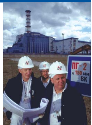
A Bechtel-led team is working on a moveable structure that will enclose the damaged Unit 4 and minimize occupational exposure for at least 100 years.
