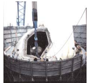
R. E. Ginna Steam Generator Replacement
