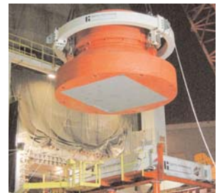
Surry Reactor Vessel Head Replacement - below budget and ahead of schedule
