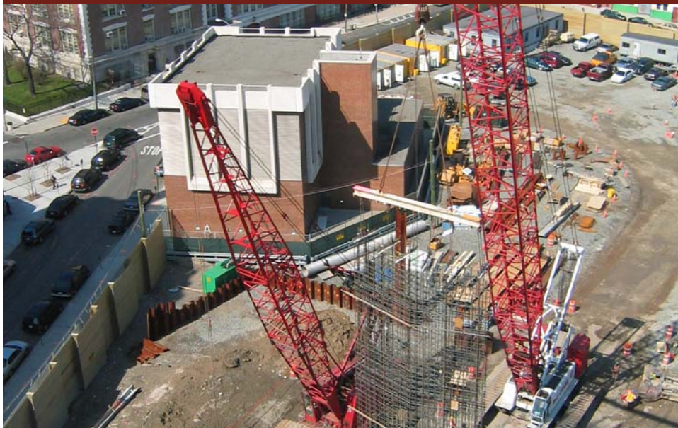
Overview of the site at Bellmouth under construction
