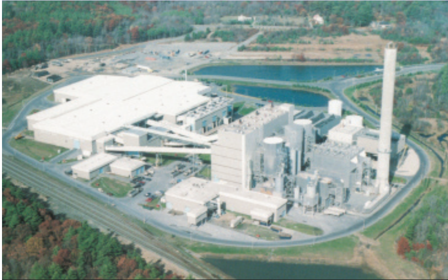
The Expansion project added capacity to the SEMASS Facility completed by Bechtel in 1989.
