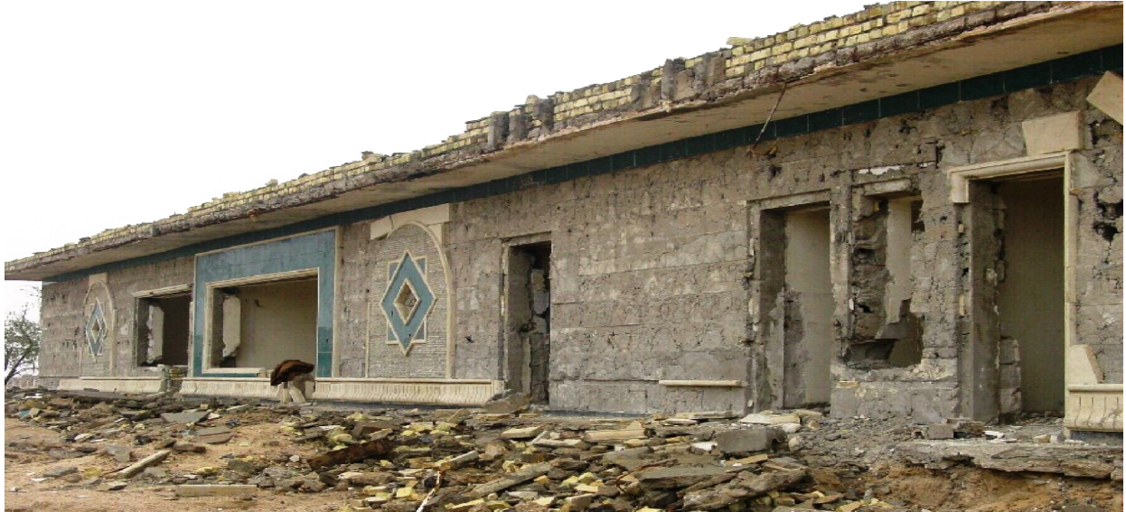
Typical Rail Station Before
