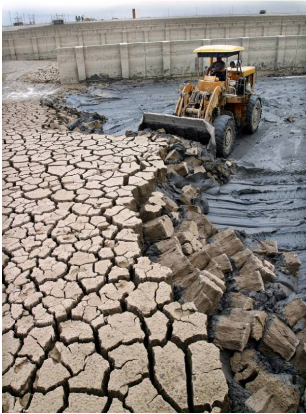
Sweet Water Canal Before
