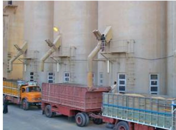
Grain Facility At Umm Qasr
