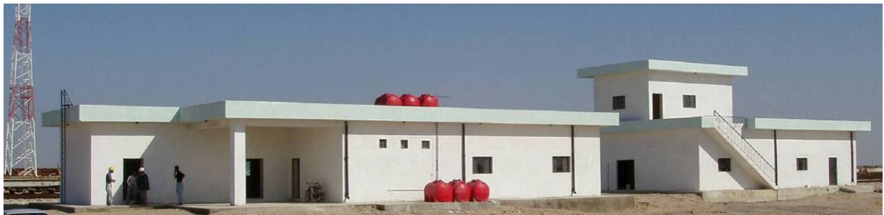
Typical Rail Station After
