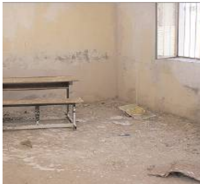
Typical Classroom Before Restoration
