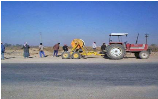
Cable Laying Along Baqubah - Khalis ITPC Backbone
