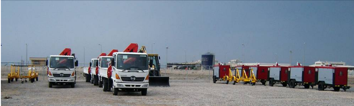
Consolidated Fiber Network Construction Equipment Delivered
