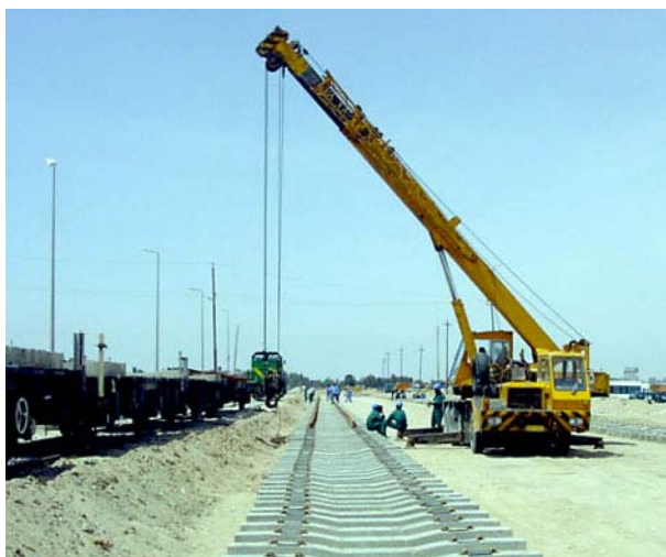
Laying New Track
