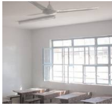
Typical Classroom After Restoration
