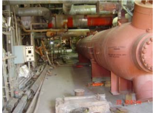
Hartha Heat Exchanger Installation Complete
