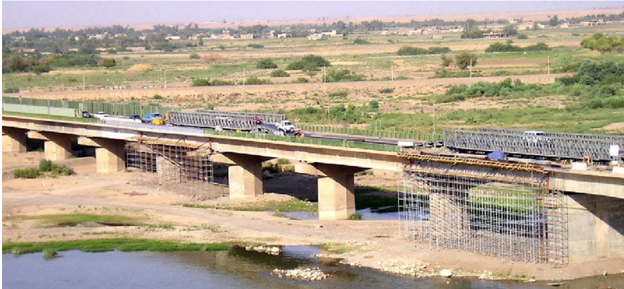
Tikrit Bridge Early in Construction
