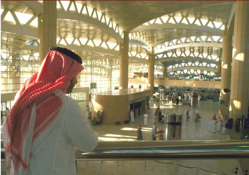
Lightweight triangular roof sheets provide the building's interior with natural light.
