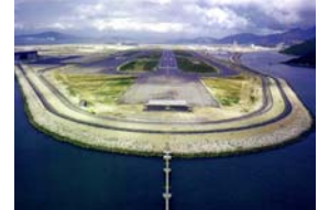
The airport site was created by flattening the island of Chet Lap Kok and adding reclamation to its western side.
