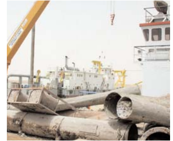
Debris (foreground) brought up from the bottom of the Port of Umm Qasr—clearly a navigational hazard
