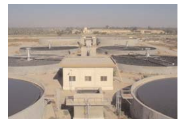
A wastewater treatment plant in operation in southern Iraq
