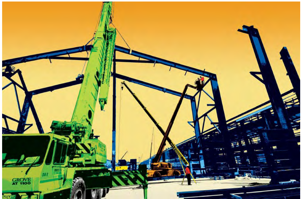
The work site at the Alba smelter in Bahrain.
