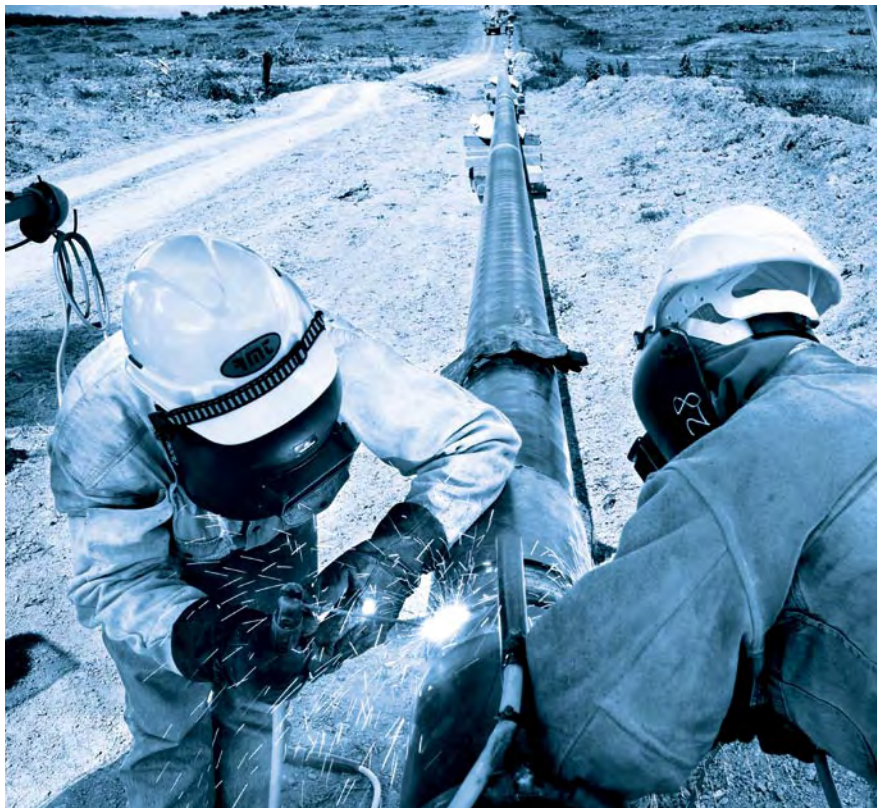
Welding on the Trans-Thailand-Malaysia pipeline.
