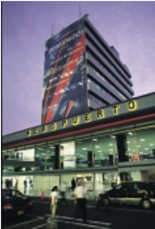
A consortium led by Bechtel Enterprises affiliate Alterra Partners is developing and operating Lima's main airport.
