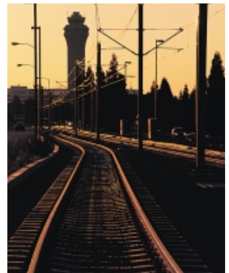
Airport MAX light-rail extension, Oregon
