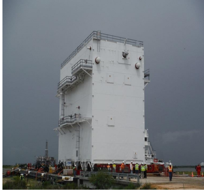
Figure 10 - Cold Boxes Delivered via SPMT
