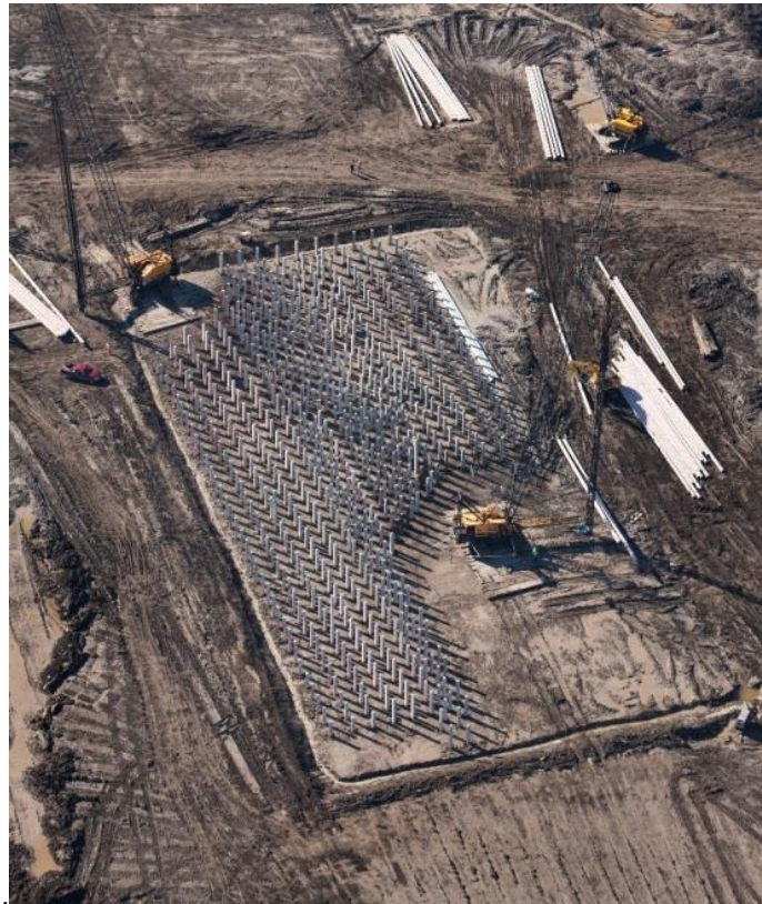
Figure 9 - Pile Driving at Sabine Pass Site
