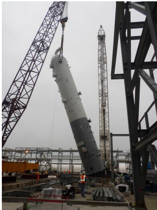
Figure 11 - Heaviest Crane Lift - CO2 Absorber
