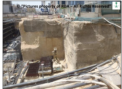
Figure 4. Soil nail support of sand backfill next to deep basement.
