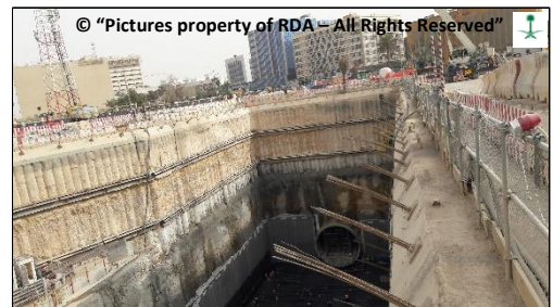
Figure 5. Anchored secant pile wall and cut in Bedded Limestone.
