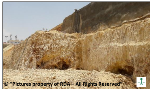
Figure 8. Typical RMP empty cavities.
