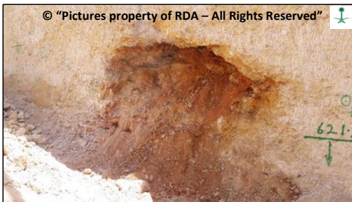
Figure 12. Infilled cavity exposing alluvial/aeolian soil (4 m width).
